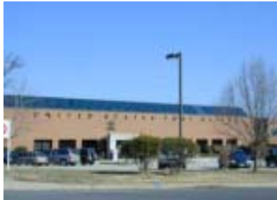
Innsbrook Post Office
